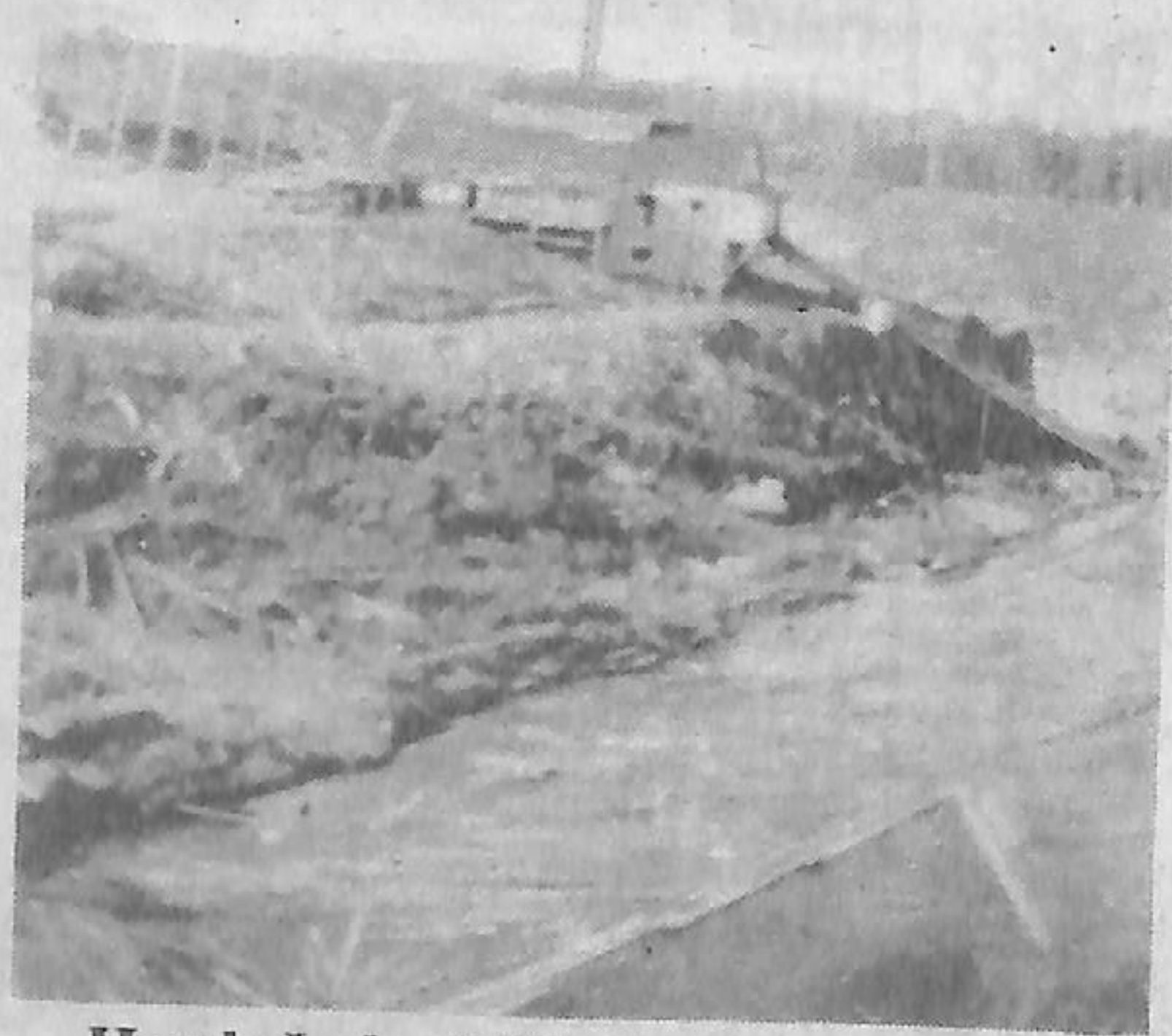
Hawk Lake Mill, along the Driftwood River in Monteith. It closed in the 1930's.
