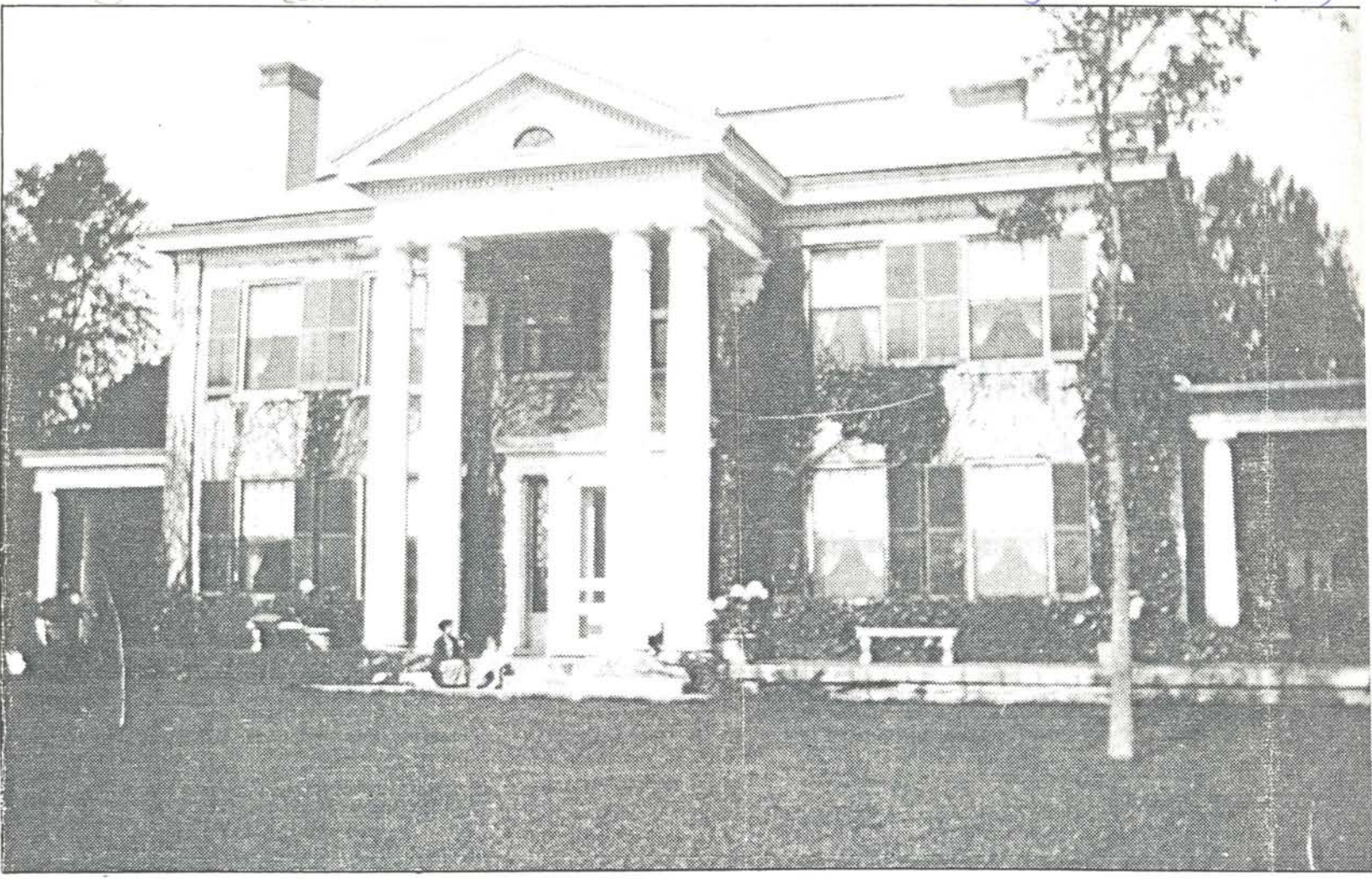
Ravensworth, circa 1910, showing the front of the house, facing the lake at the bottom of Fitzhugh Lane. The house looks similar today.
