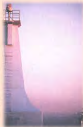
Cobourg Lighthouse East Pier
