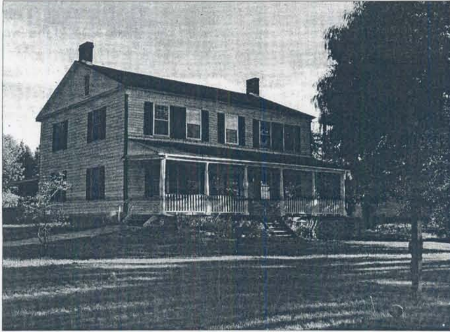
The former Rose Lane Inn once comforted travellers making the trip from Toronto to Kingston. The inn has seen a lot of owners but little has been done to take away from the heritage look of the building.
