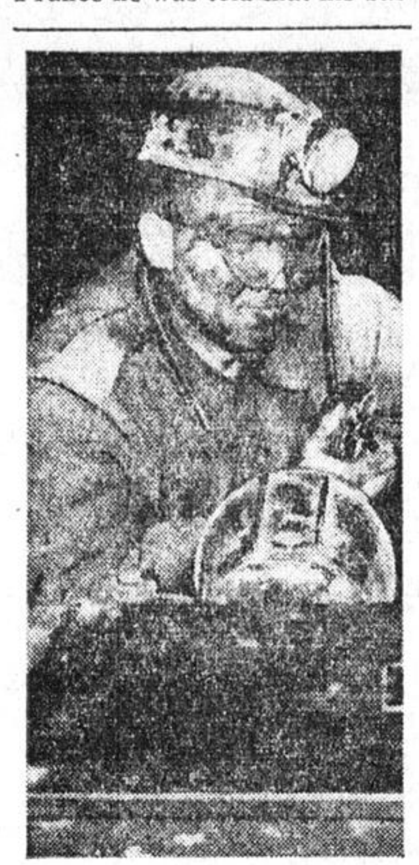
In the undersea coal mines of Cape Breton, N.S., coal trains are often equipped with two-way radio phones to assure constant communications with the surface.
