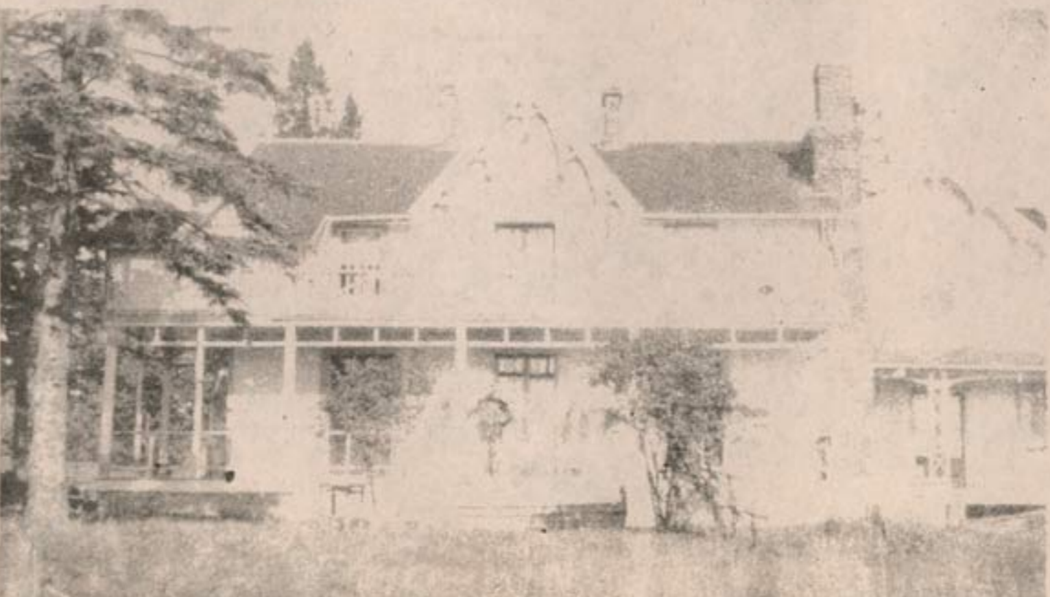
Quorn Cottage, picturesque neighbor of Kelwood.
