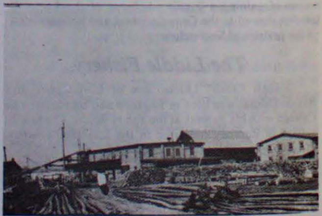
Crewe Bros. fishery showing their large supply of poles used for their pound nets. Piles of bolts 38 feet long are ready to be cut into 1/2 inch lumber for fish boxes.
