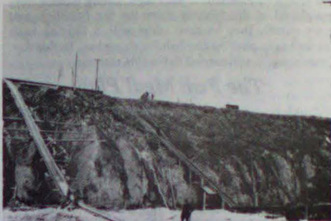
Crewe Bros. fishery: A scene of the ice harvesting operations. The four-wheeled "donkey" is conveying the cakes of ice up the 78 foot bank.
