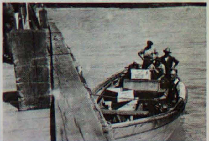
An Omstead - Furey crew at the dock in the 1920's.
