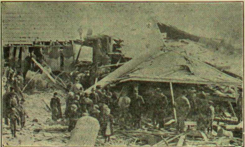
The Town's Second Boiler Explosion, April 6th, 1896—Watson Brothers Heading Mill
