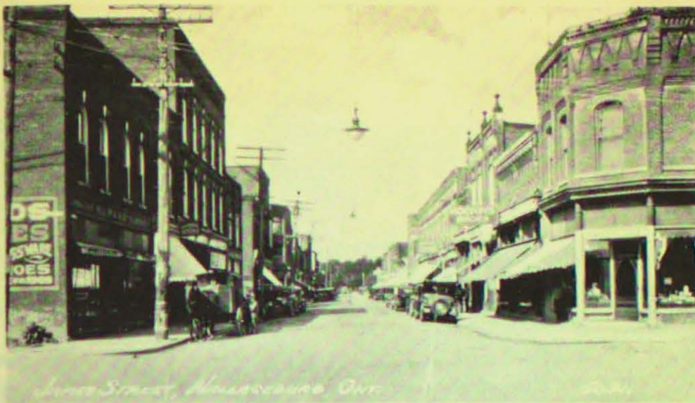
JAMES STREET LOOKING WEST FROM NELSON STREET - 1937.
