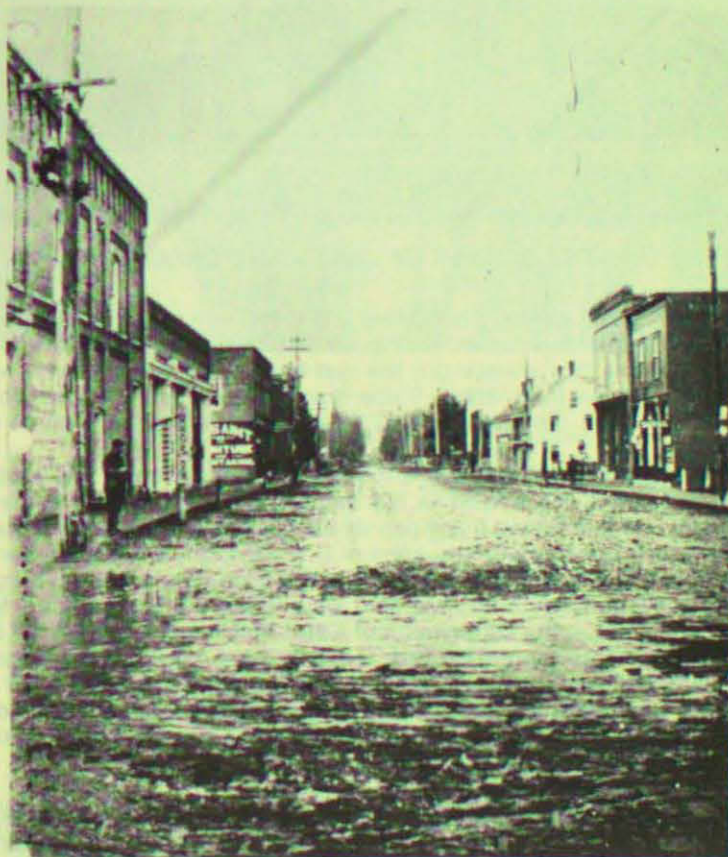
NELSON STREET LOOKING NORTH FROM JAMES BEFORE PAVING IN 1902.
