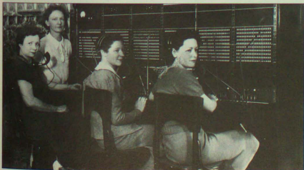
NUMBER PLEASE? Hundreds of occasions each shift, that phrase was routinely uttered by Wallaceburg Bell telephone switchboard crew, who were stationed at the phone centre on Duncan Street, opposite Knox Presbyterian Church. This 1930s Bell crew shows Anne McLean standing with Mrs. C.R. Gormely, Kate McPhail, and Jessie Barnes at the switchboard. (Mann Historical Files.)
