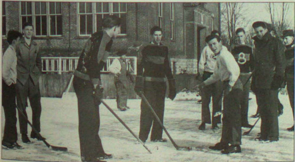
RINK RATS OF '44. The outdoor hockey rink at Wallaceburg High served well during the pre-arena days. There were always eager volunteers to erect the boards and flood the ice as long as boiler room warmth was provided. Here, a group of high school seniors stage an informal game of shinny, although the goalie is not quite ready! In background, Francis Benninger is strapping on his goaltenders gear. Ready for play are Joe Taylor, Jim McKenzie, Jack Glendinning, Jay Richardson, Andy O'Flynn, John Jae (No. 8), Bob Jordan, and Andy Truan. (Roy Mathany Photograph.)
