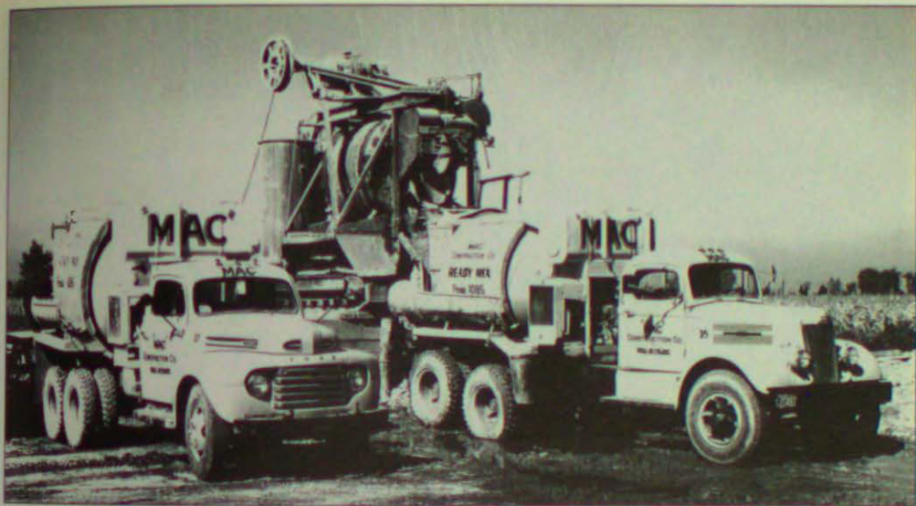
TWO BIG MACS. That did not mean hamburgers when this scene was photographed during the 1950s. Founded by Eric MacDonald in 1944, Mac Construction Company became a leading building contractor in Western Ontario, the firm later managed by second generation member Dean MacDonald. The pictured Mac Construction Ford and White cement mixers were resplendent in their bright yellow paint exteriors as they carted mixed concrete to the various building sites. (Wallaceburg Museum Collection.)
