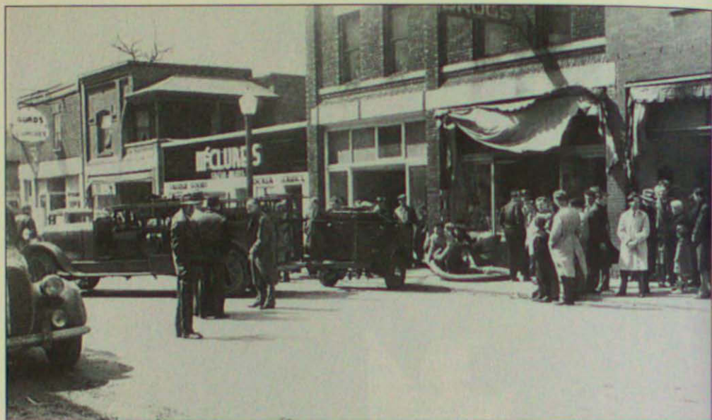
DOWNTOWN HOT SPOT. Fortunately there was little damage in this 1946 James Street scene when a call reported a fire at Archie Vivian's Drugstore. The venerable 1929 Reo hose and chemical truck was on the scene in a matter of minutes responding to the alarm. That huge ice cream cone marks the site of Pop Gurd's sweet shop, with other locations including Paul Pollock's Men's Clothing, Gord McClure's Frozen Food Lockers, Smith's Hardware, and Douglas-Haycock Furniture, right. (Mann Historical Files.)
