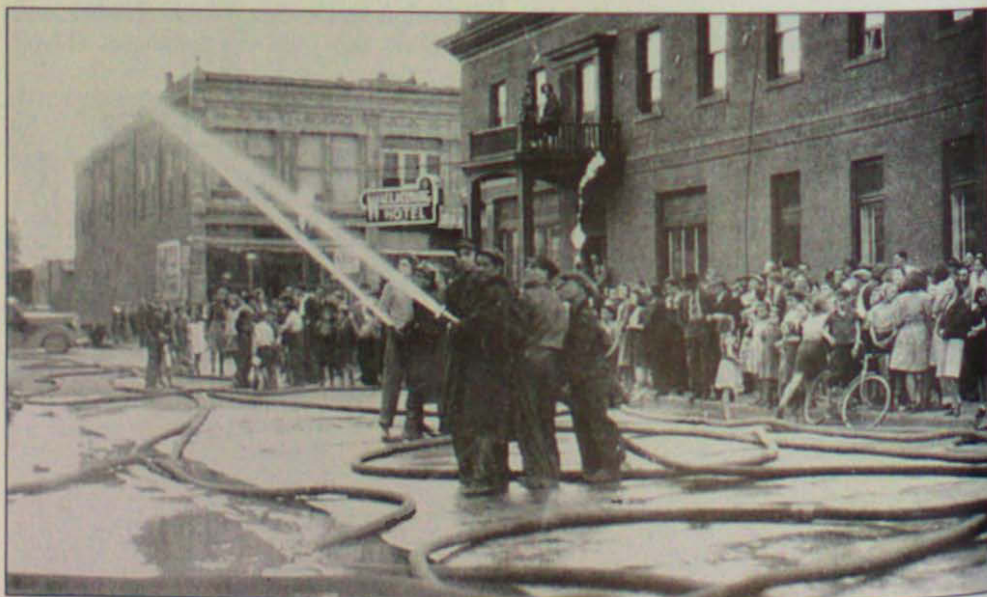
ARLINGTON AIM. Volunteer members of the Wallaceburg Fire Department train their hoses on the flames at the vacant Arlington Hotel on Wallace Street during an April 29, 1942 fire. A large crowd gathered to watch the vacant structure experience its final hours. (Roy Mathany Photograph.)
