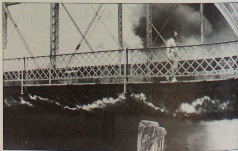
HOT COALS PUNISHMENT? With Central Bridge in flames, local druggist Frank Nightingale seems to be taking a casual stroll over a bridge barbecue. In fact, Frank is running for dear life, hastening to return to his McDougall Street drugstore in this spectacular 1944 inferno. (Mann Historical Files.)
