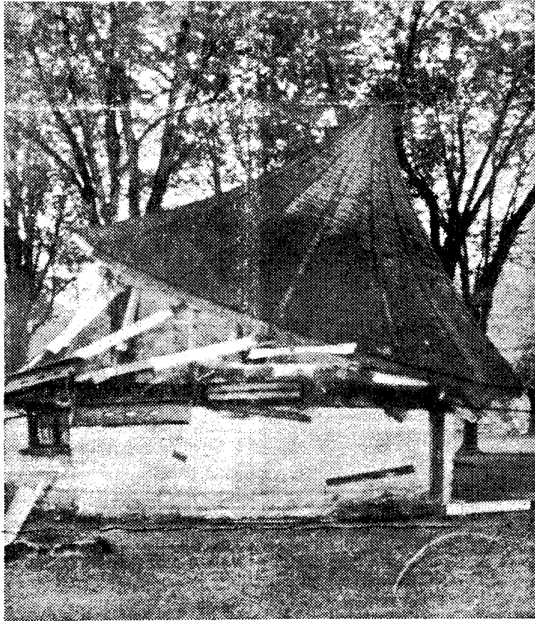
The old band stand in Victoria Park was pulled down about seven years ago by tractor and cable. Three pulls were required to bring the structure to the ground.
